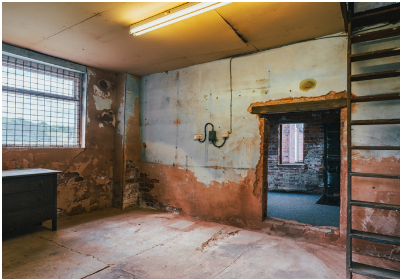
STORE 1 & VIEW INTO STORE 2
