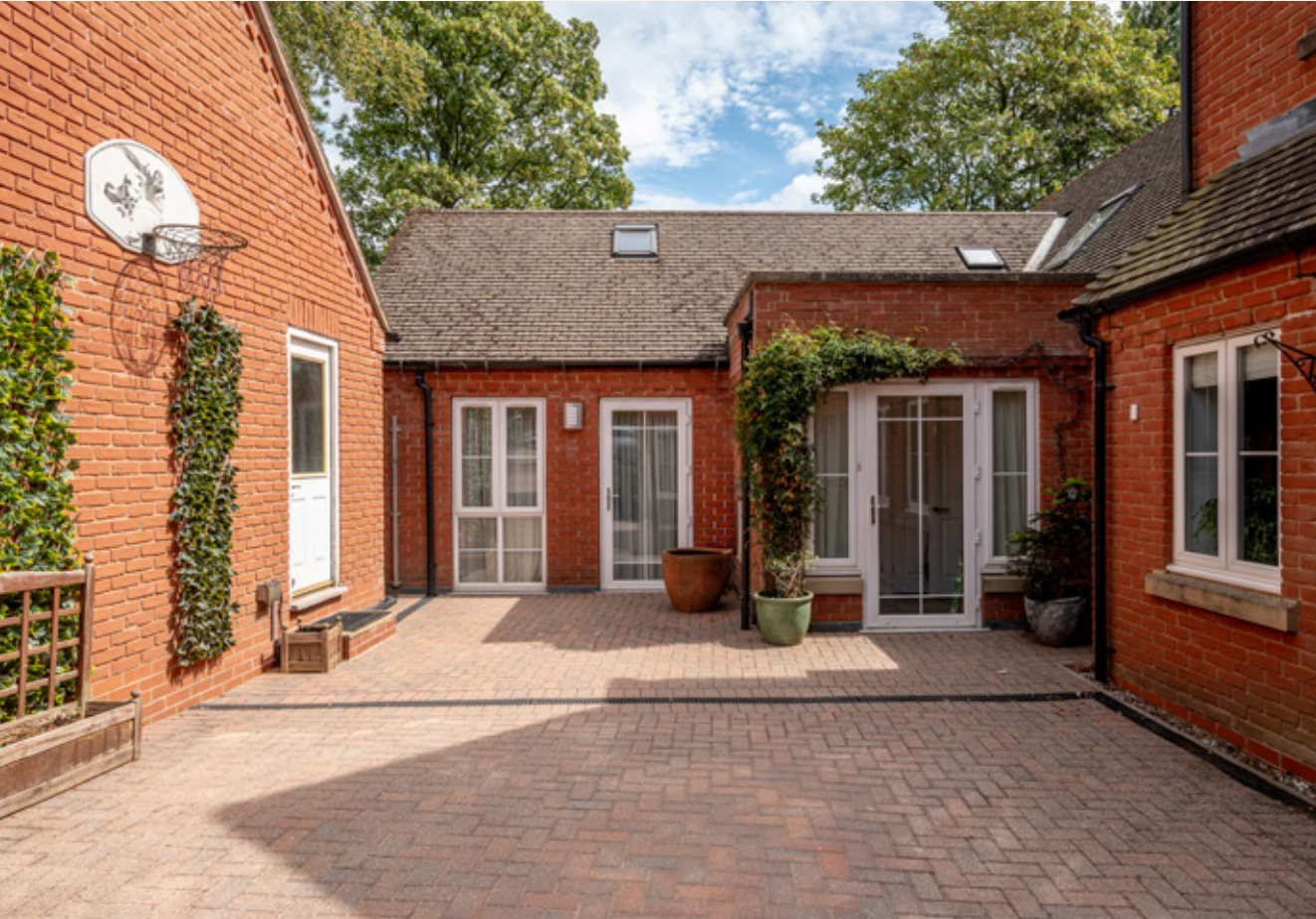
FRONT OF SELF-CONTAINED ANNEXE
