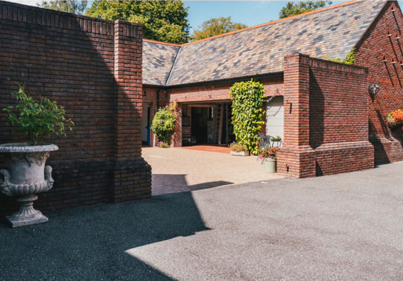
COURTYARD LEADING TO GARAGING & WORKSHOP WITH GARDENER'S WC
